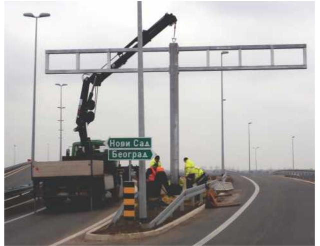
Cantilever production and installation
