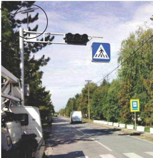
Pedestrian crossing signal with lantern and three illuminated running pedestrian figures powered by solar panels
